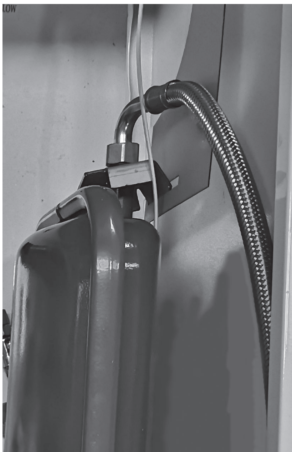
Figure 4-2: Expansion vessel, Expansion vessel bracket and hose connection - System model only
