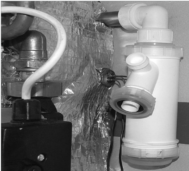
Figure 6-2: Condensate trap
