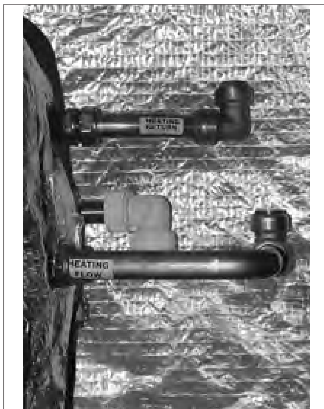
Figure 5-1: Non system boiler flow and return connections
