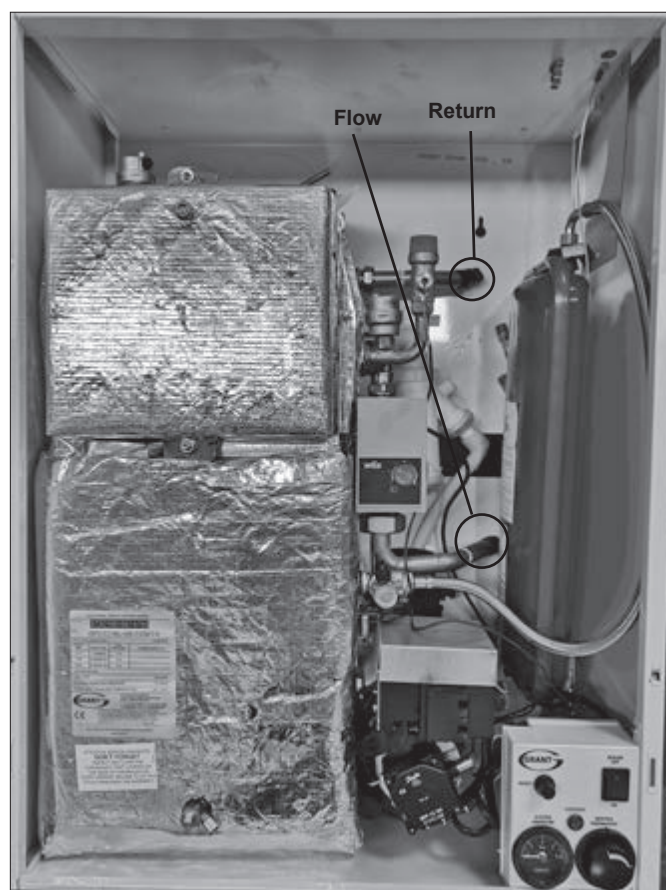
Figure 5-2: System boiler flow and return connections
